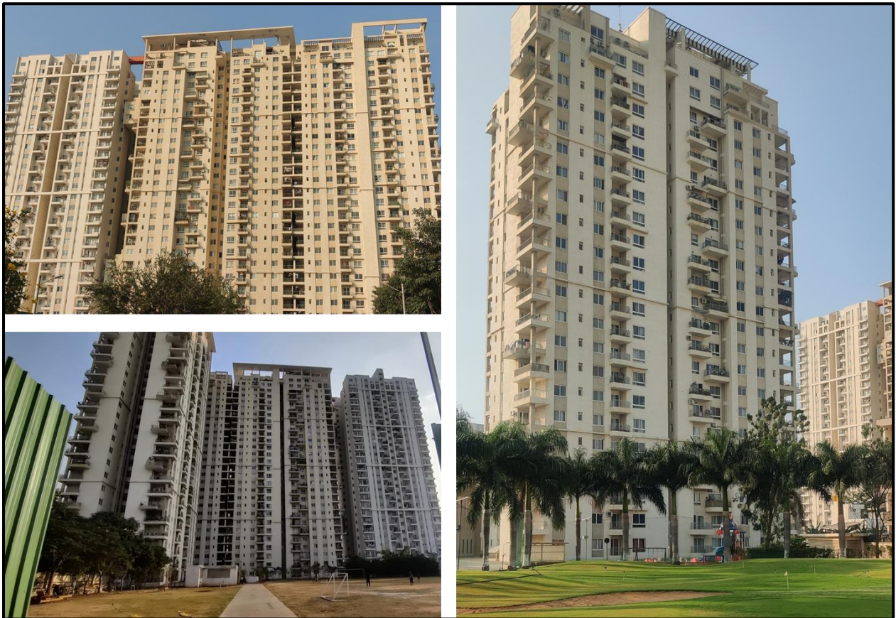
Photos: Completed Blocks of the Project
