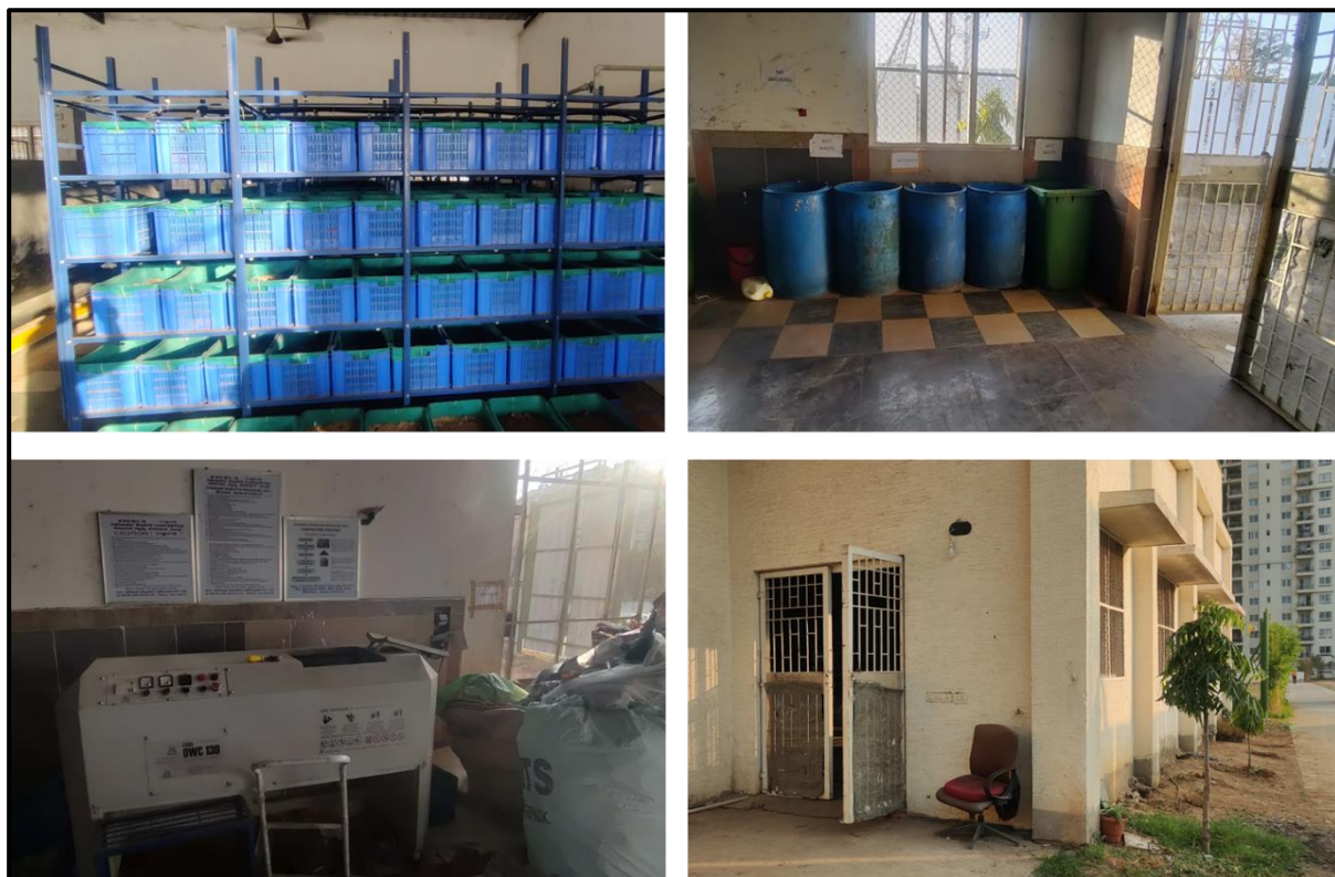
Photographs: Solid Waste Management Facility at Project Site
